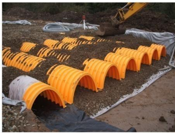
Please ensure before back filling that isolator row is completed as per instructions.
