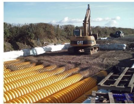
10. Backfill chambers to required depth as per attached drawing.
