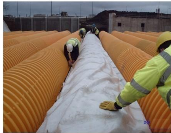
7. Wrap isolator row with supplied filter geotextile, ensuring that the holes at bottom of chamber are covered completely. Use only supplied filter geotextile
