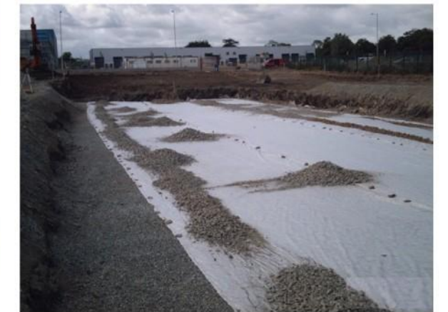
11. Lay supplied geotextile over final layer of stone
