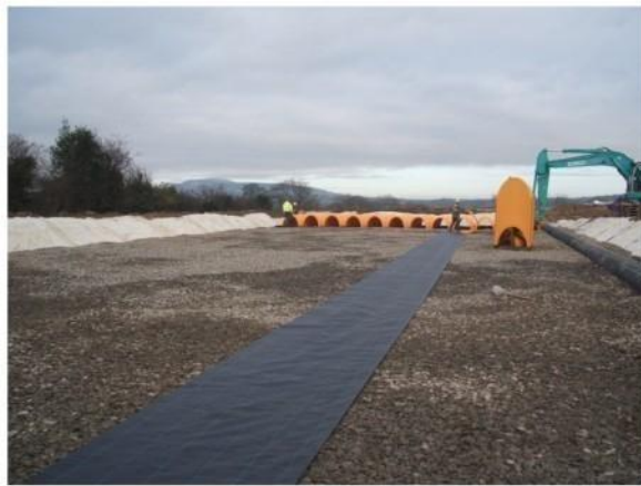
7. Place black geotextile under isolator row. This will be shown as a shaded row on attached drawing.
