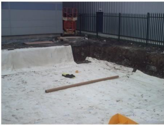
1. Dig excavation. 2. Line base and walls of excavation with supplied Geotextile. 300mm overlap required on all Geotextiles.
