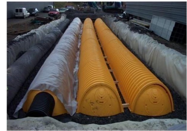
8. Cut required hole in endcap. Connect supplied pipe from chamber to manhole. Pipe will enter manhole at chamber invert level.
